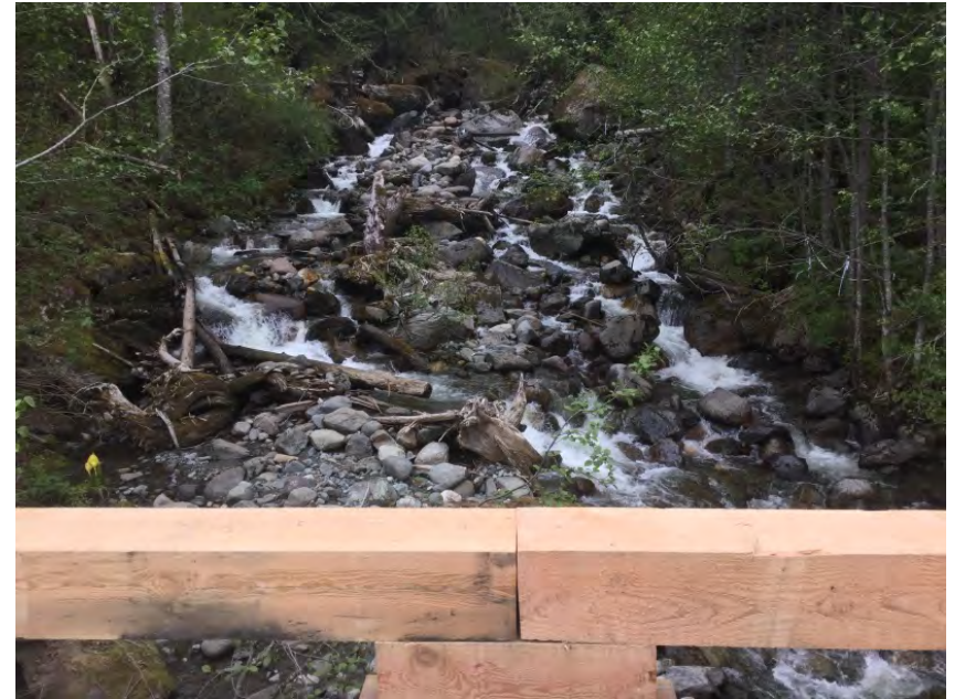
Upstream from Crossing
