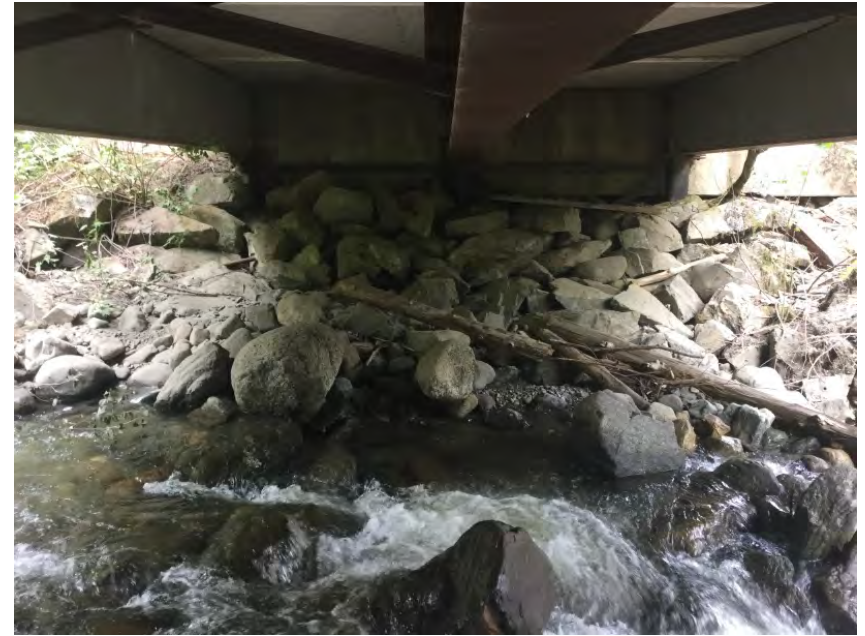
Left Bank Abutment when facing downstream
