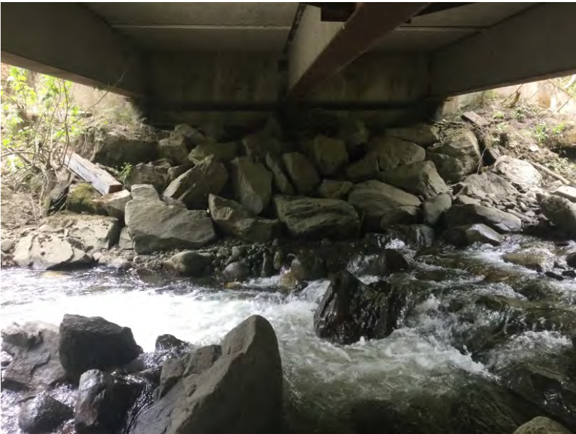
Right Bank Abutment when facing downstream
